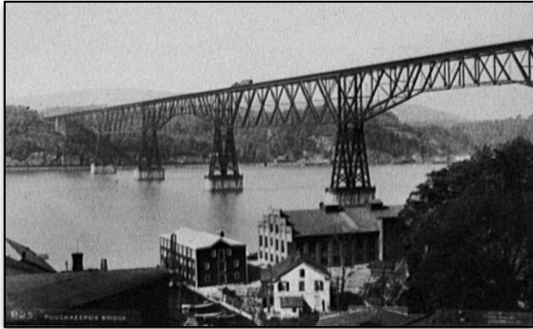
When it burned in 1974, the loss of the Poughkeepsie Railroad Bridge dealt a major blow to Orange County's remaining railroads. The bridge is now used as the Walkway Over The Hudson (Library of Congress).
